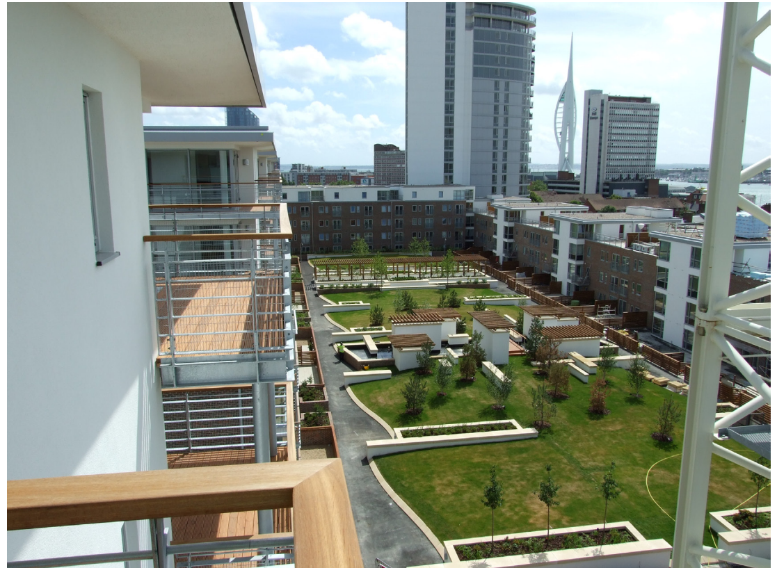
A view looking south across the rooftop gardens of Admiralty Quarter, with the Spinnaker Tower in the distance
