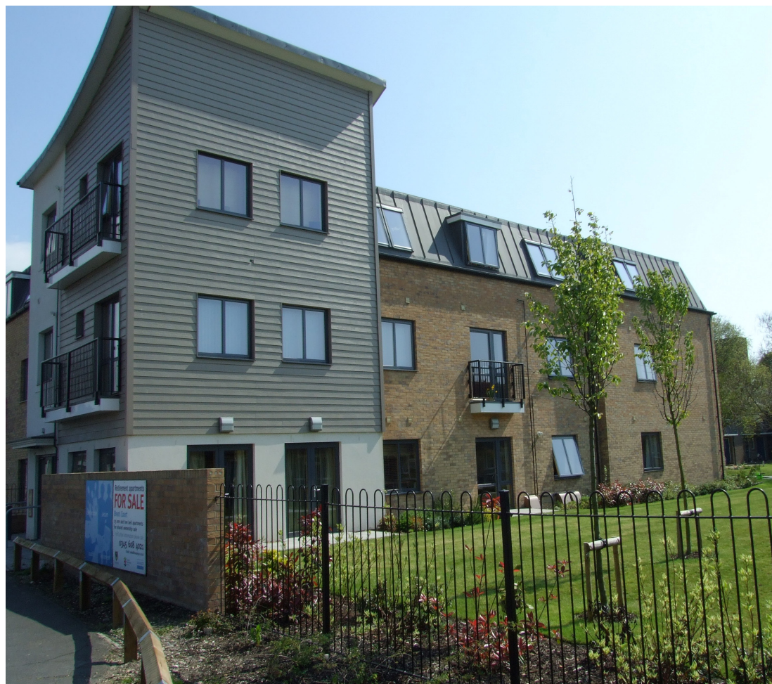
The Milton Village development, Portsmouth: an extra-care mixed-tenure scheme with 62 flats developed in partnership with Housing 21, completed late 2010. One third of the flats are shared ownership and two thirds social rented
